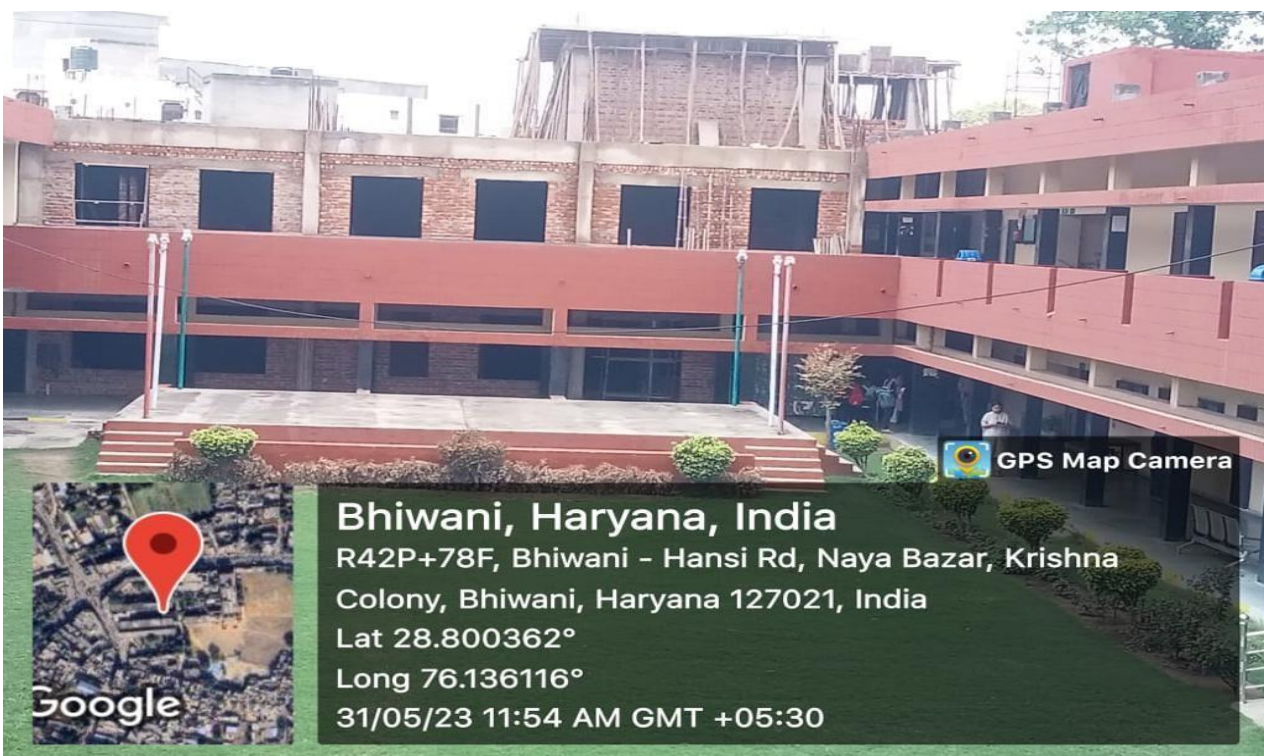
New Library (Under Construction)
