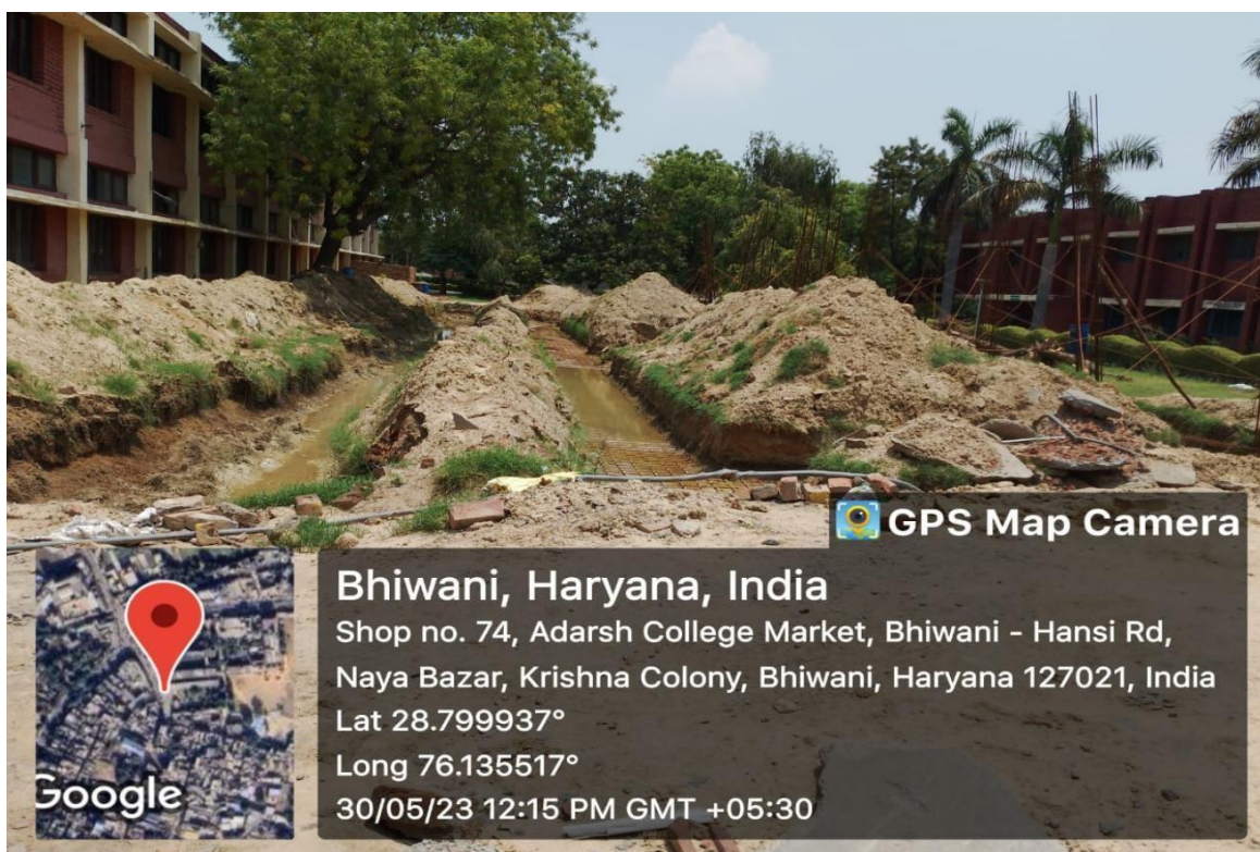
New Science Block (Under Construction)
